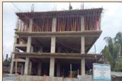
10-Storey Hospital Under Construction Likely to be completed by December, 2024
