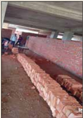
Construction on Progress
